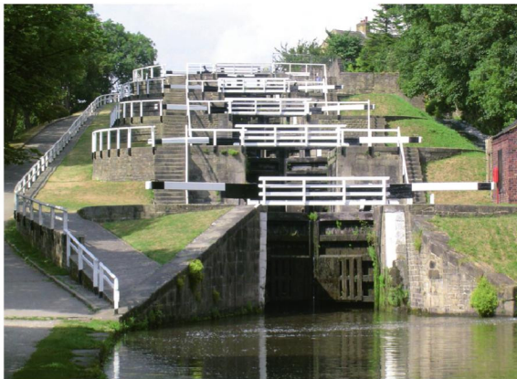
Bingley Five Rise is perhaps the best-known set of staircase locks on the system.
