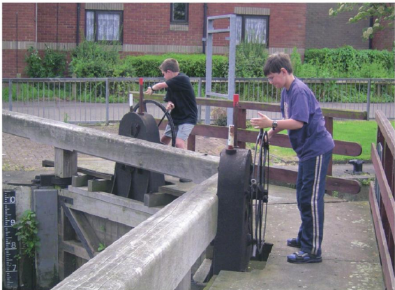
If necessary, the electronic locks on rivers can be operated manually.
