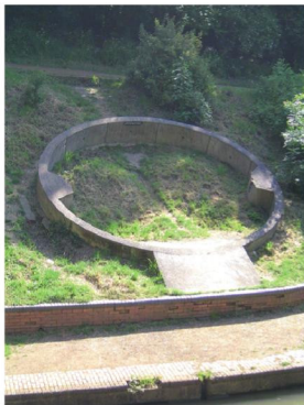
A section of the lining used to restore the Blisworth Tunnel.
