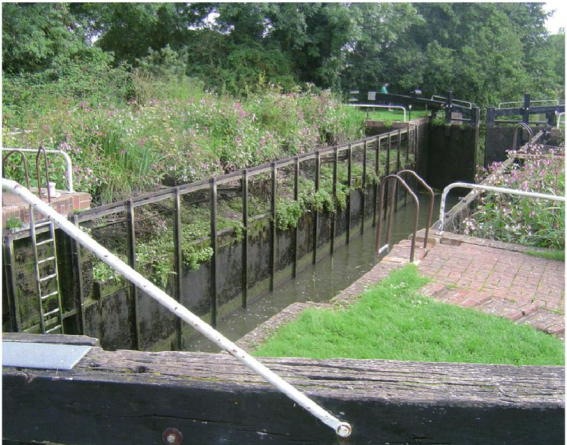
Monkey Marsh Lock on the Kennet & Avon, a rare example of a turf-sided lock.
