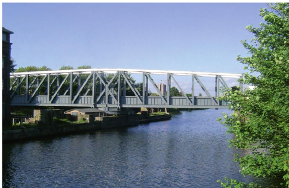
The 'modern' Barton Aqueduct is an impressive swing bridge which moves with the water inside it.
