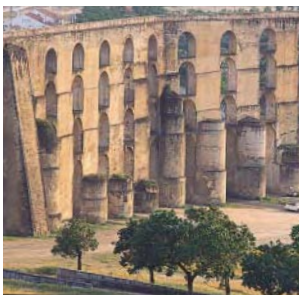
Aqueduct between Amoreira and Elvas
