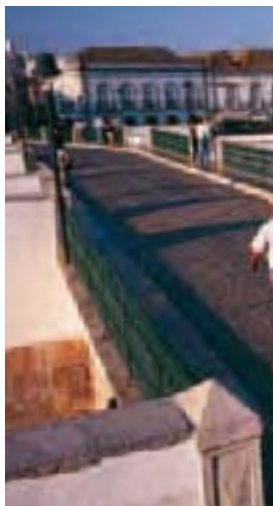
Roman bridge (Ponta Romana)
